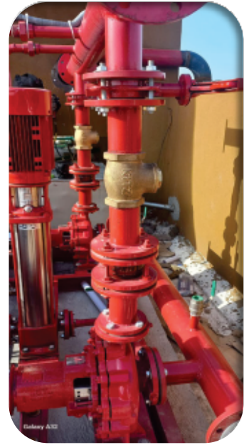
Installation of Fire fighting pump at Panaghah, Tarlai, Islamabad
